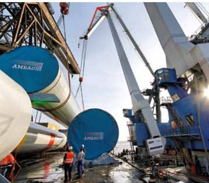
Loading of offshore tower segments
