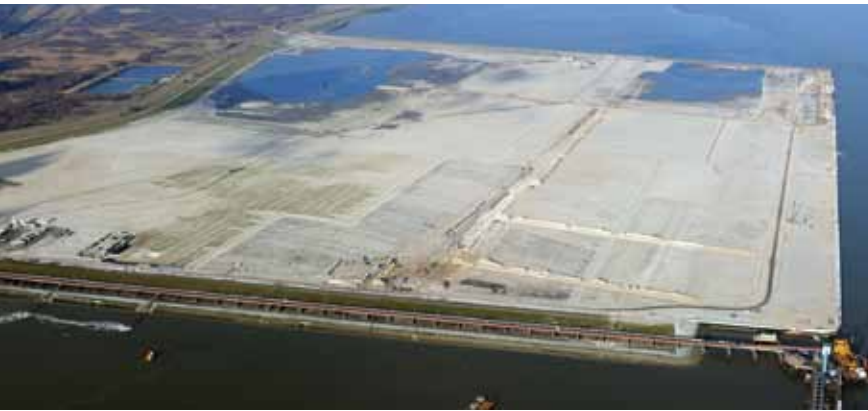
Construction work on the EUROGATE container terminal in Wilhelmshaven is proceeding rapidly.
